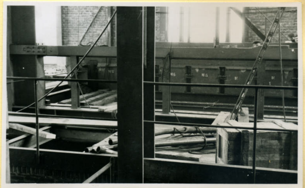
Ketel 0. Montage rooster.
