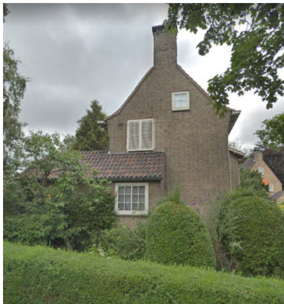
Provincialeweg 250 – Street View 2018
